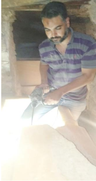
Fig. 7 During drilling in the first part
