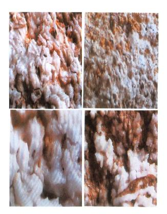
Due to the continuous crystallization and recrystallization of these hygroscopic salts inside the limestone blocks, these blocks have become seriously exfoliated, fragile, and incohesive.
