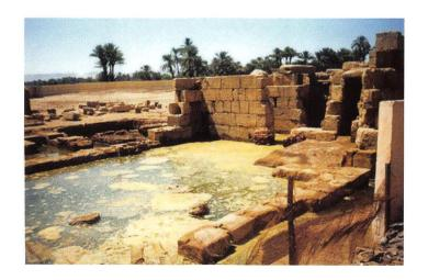
The colonies of various microorganisms (mainly algae and fungi) have been extensively scattered on the limestone blocks used for building the Cairo walls in 11th century. These microorganisms have contributed greatly to the deterioration of mineral constituents and the structure of these stones.
