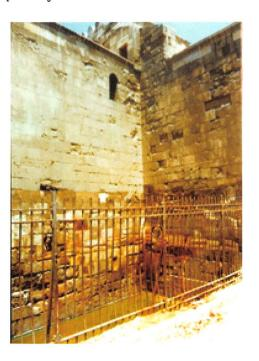
The absorbed saline solution is the main source of the crystalline salts, which form a thick hard crust on the walls of these buildings.
