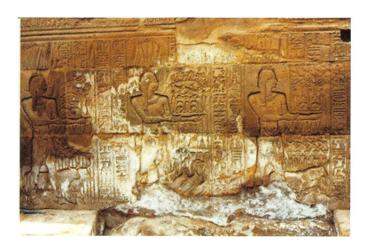
On the other hand, rain water penetrating into the monumental limestone causes the dissolution of its mineral constituents, and transports the mineral constituents to the surfaces of these stones to develop a hard crust of these minerals mixed with salts that readily produce a very common deterioration phenomenon which is called "honey comb" weathering.
