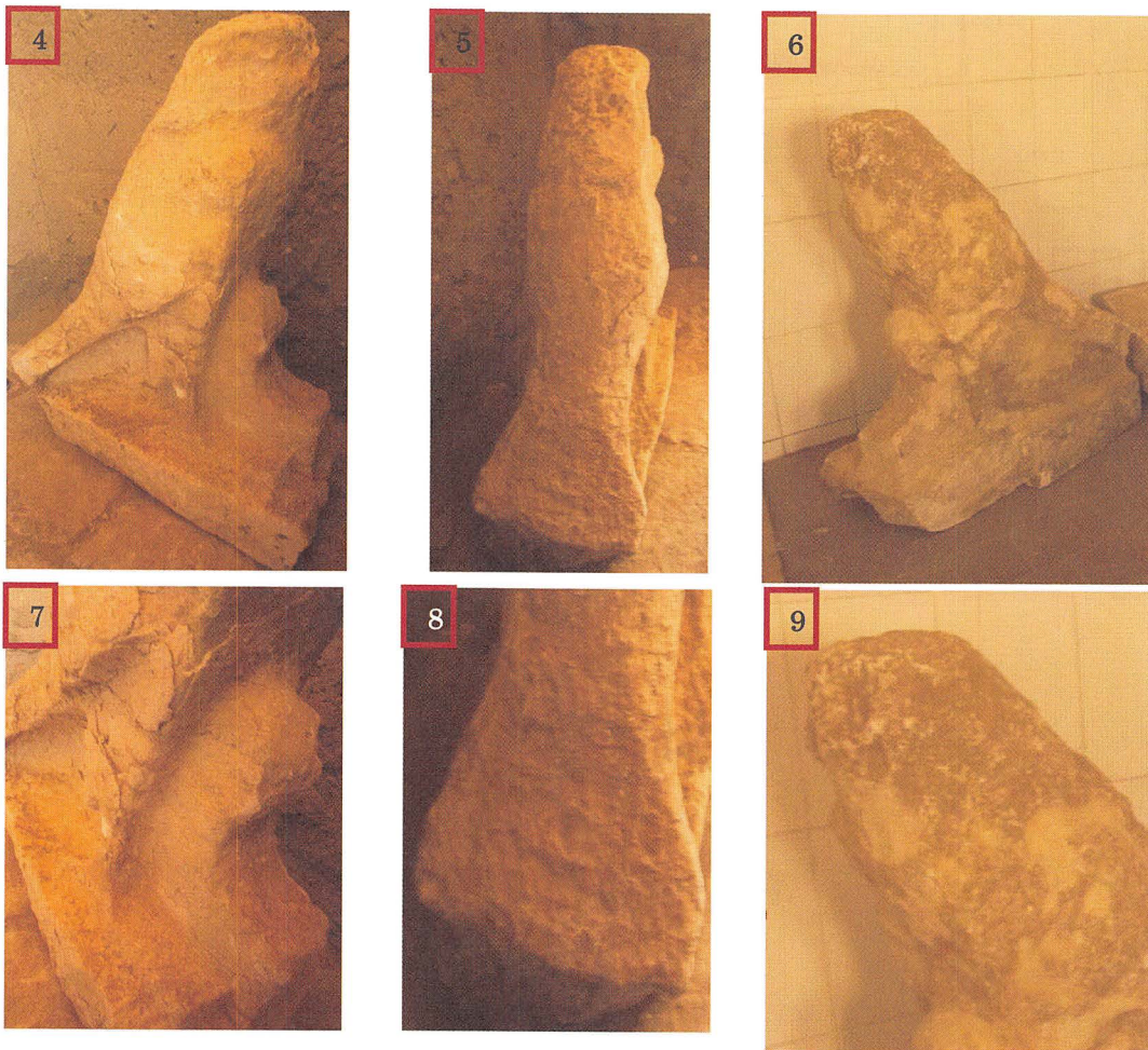
Figs. 4-9 The deterioration on the statue of the falcon, flaking, the sand and salt that covered the surface, and the surface erosion
