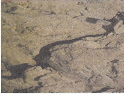
5) Mechanical cracks along the galleries
