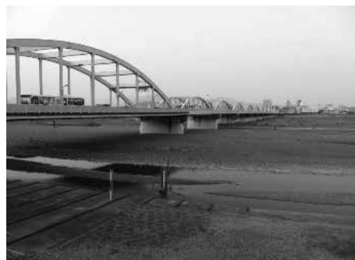
Fig 17. Akekawa River bridge
