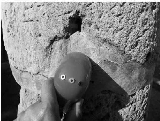
Fig.13 No.5 block (Repaired part)
