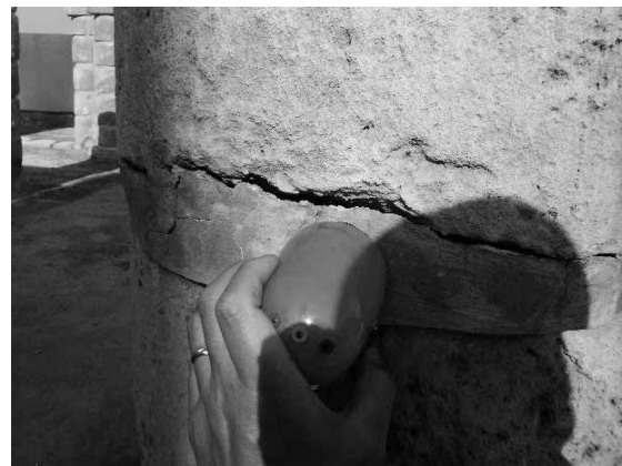
Fig.14 No.6 block (Repaired and stripped part)
