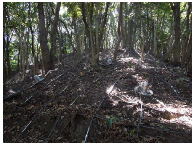
Figure.1 Example of construction
