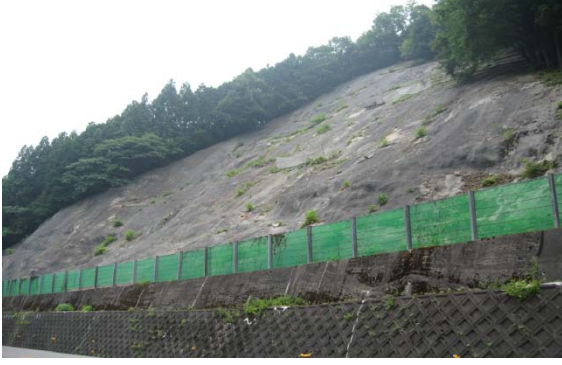
Figure 2. View of the shotcrete slope (A-district)
