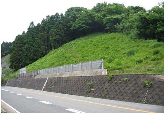
Figure 3. View of the non-support slope (B-district)
