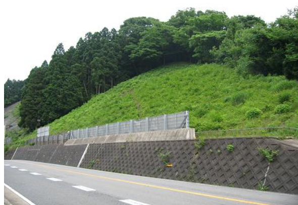
Figure 3 View of the non-support slope (B-district)
