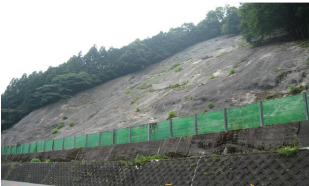
Figure 2 View of the shotcrete slope (A-district)
