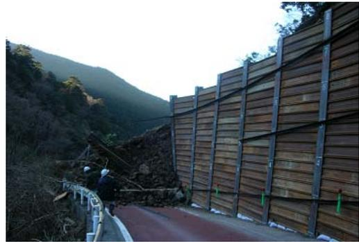
Figure4. The circumstances of failure
