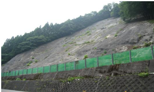
Figure.2 A large-scale slope covered shotcrete. (district A)
