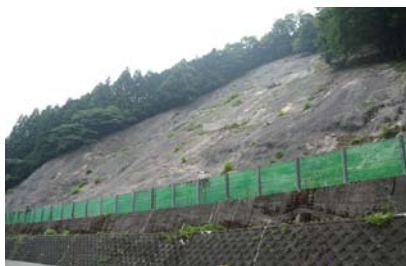
Figure-2. View of the shotcrete slope (area-A)
