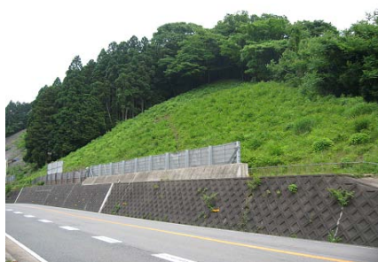
Figure-3. View of the non-support slope (area-B)
