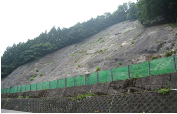
Figure 2. View of the shotcrete slope (A-district)
