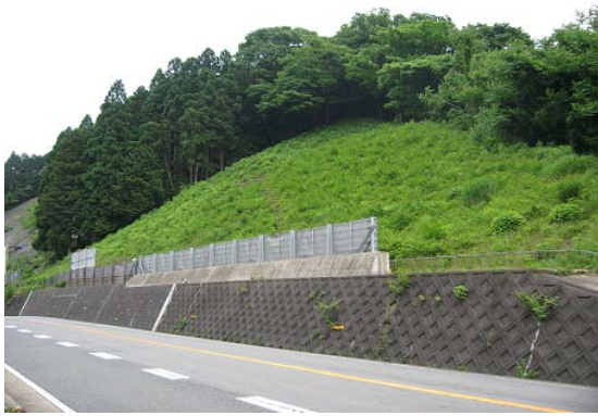
Figure 3. View of the non-support slope (B-district)
