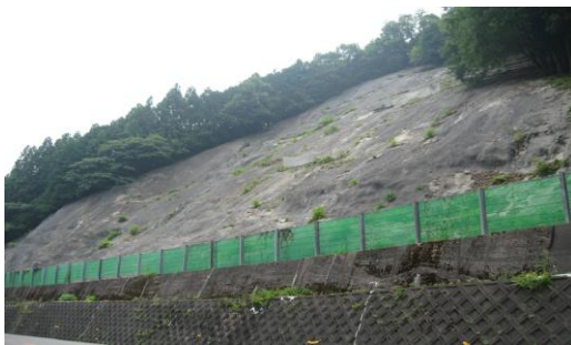
Figure.2 A large-scale slope covered shotcrete. (district A)
