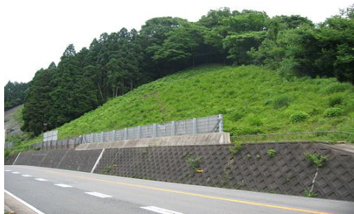
Figure.3 A small-scale cutting ground slope. (district B)
